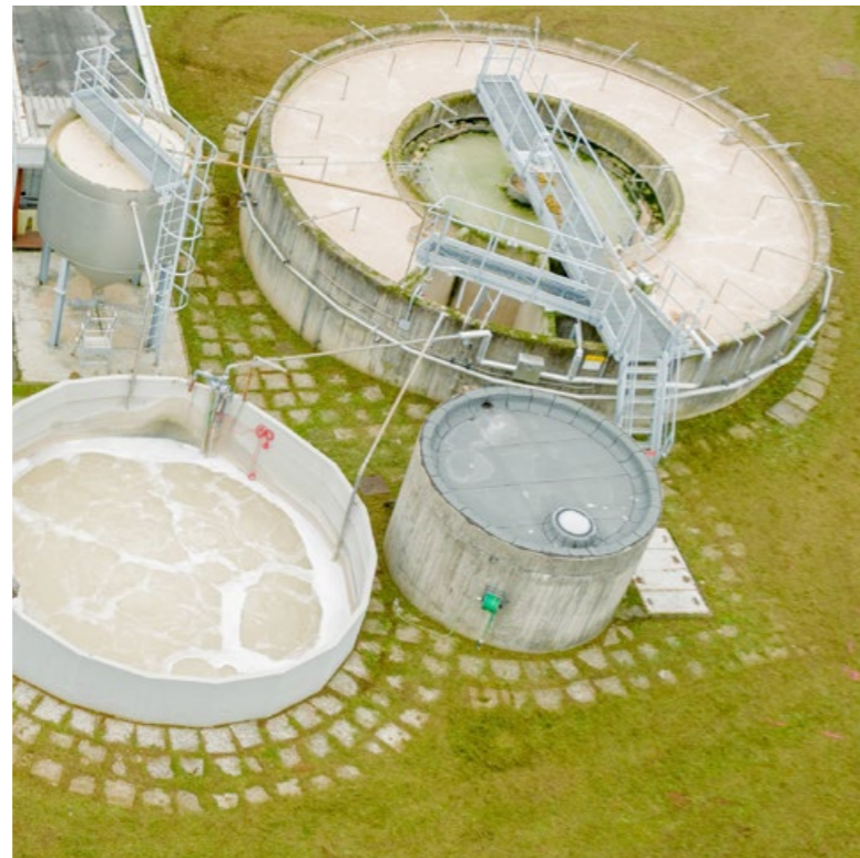
Wastewater treatment plant Origgio Site
